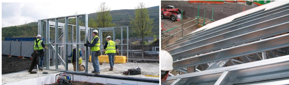
Installation of light steel wall panels and roof trusses
