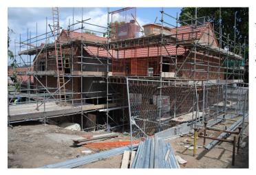
The Frame and boarding out of the structure took just over 6 weeks to erect which then allowed for the external finishes, roofing etc. to be applied.
