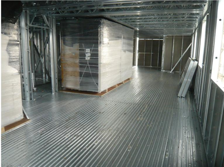
Givlon screed. Despite the increased weight, relative to a timber alternative – 22mm plywood – the stiffness gained and ‘improved feel’ of the finished floor with improved build speed are a significant factor in the project. In some cases, a combination of load and span, the Givlon screed and Lewis deck can also give increased clear spans of the lattice trusses for a given depth of floor construction.
