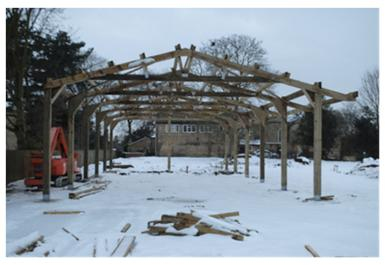
The structure comprised of a main workshop with smaller subdivided stores and a boiler room. With typical bay widths of 4.572m
