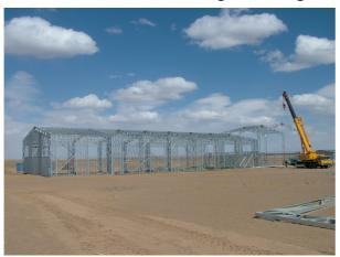
between the timber deck and the top chord of the light gauge steel trusses. Deflection, and design checks, in accordance with SCI P301.
